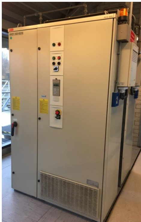
Figure 15. ACS607-320-3 cabinet drive on client site and internal layout with R9 inverter module For the ease of setting up and designing the frame solution, all components should be fitted into one section of the cabinet. Another critical task for the new design, apart from updating components for the main circuit, is to enable the installation and use of lot of other electrical
