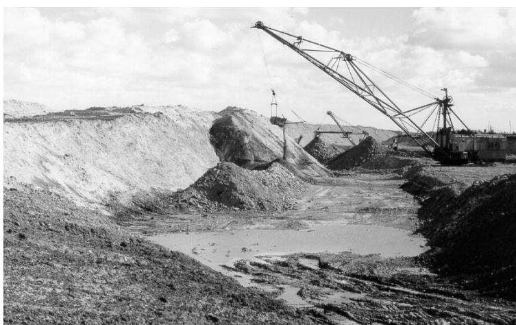
Fig. 7. Pit at the end of the trench before 1997. Limestone pile on the bottom of the trench forms under spoil drainage channels
