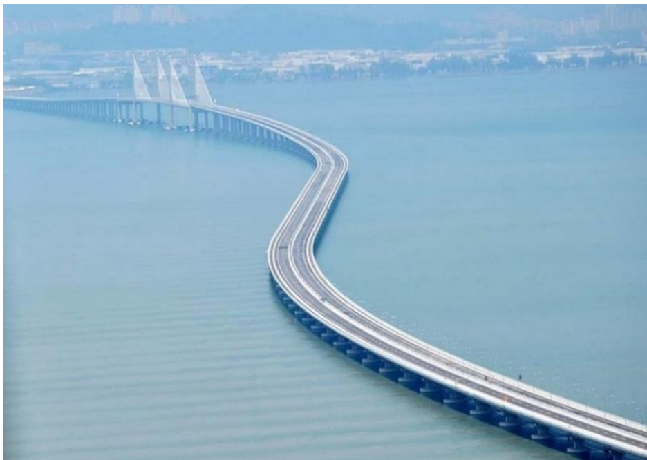
Foto 7 - Second Penang Bridge [20]
