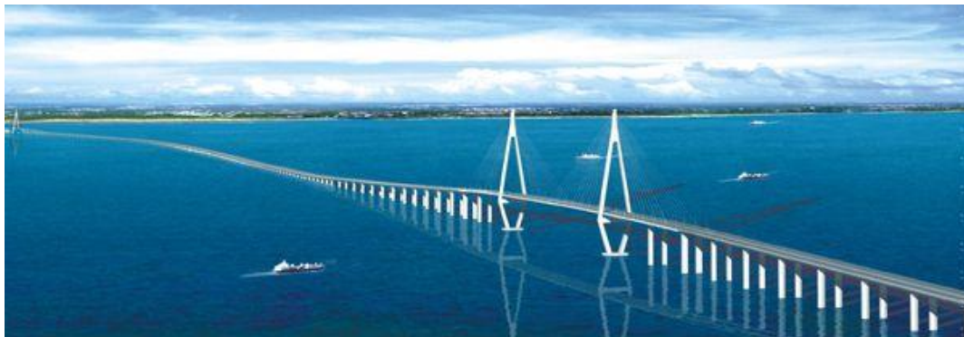
Foto 5 - Hangzhou Bay Bridge [8]
