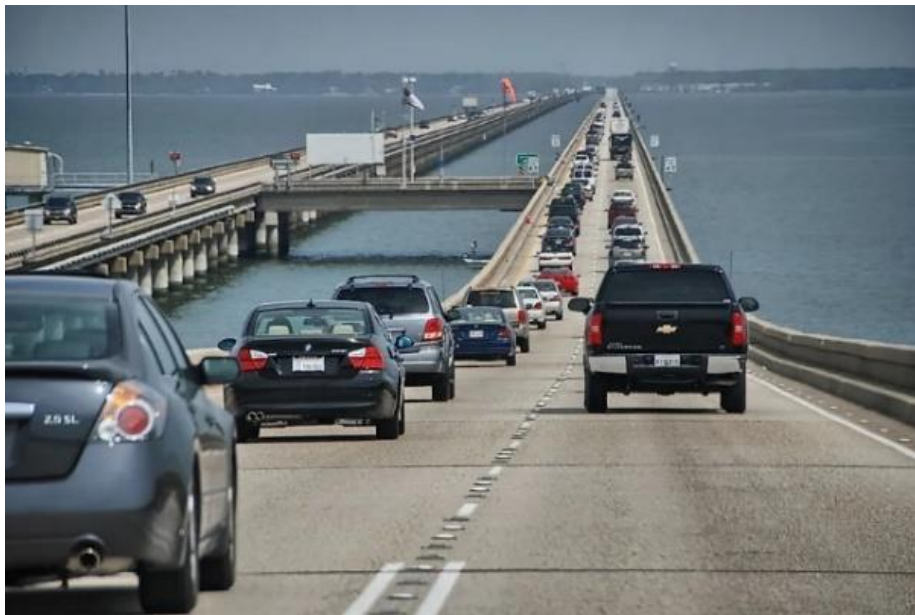
Foto 8 - Lake Pontchartrain Causeway Bridge [7]
