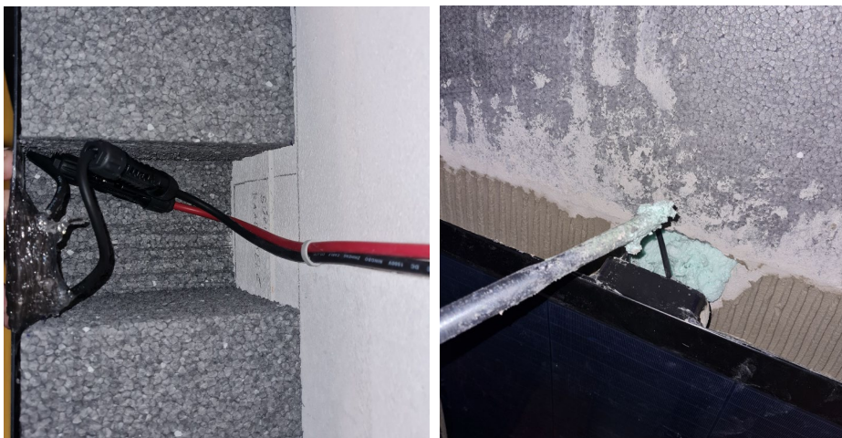
Figure 11. MC4 connectors in cavity during demo application before insulating the whole facade (left) and filling the cavity during the application of PV panel (right). Lengthening cables between PV panels are attached to the AAC structure and would stay in place even after replacing the PV panels.
