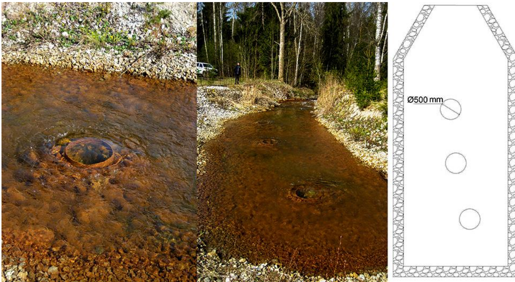
Figure 11. Ahtme three overflow boreholes and a visualized scheme of the boreholes. (Photos taken in 17.05.2017 by S. Lind)
