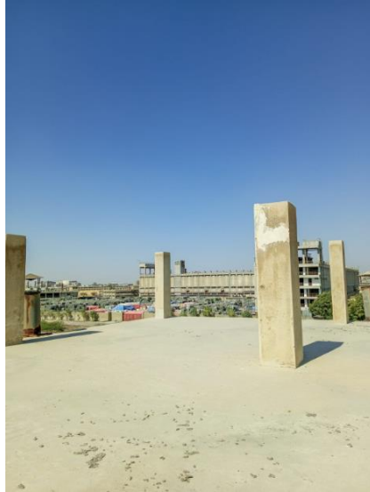
Figure 4.6 View of roof top
