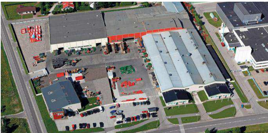
Figure 1 Fors MW AS plant in Saue (FORS MW, 2021)
