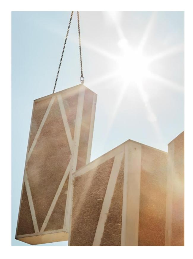
Figure 7. Ecococon wall system. Source – Ecococon, 2021
